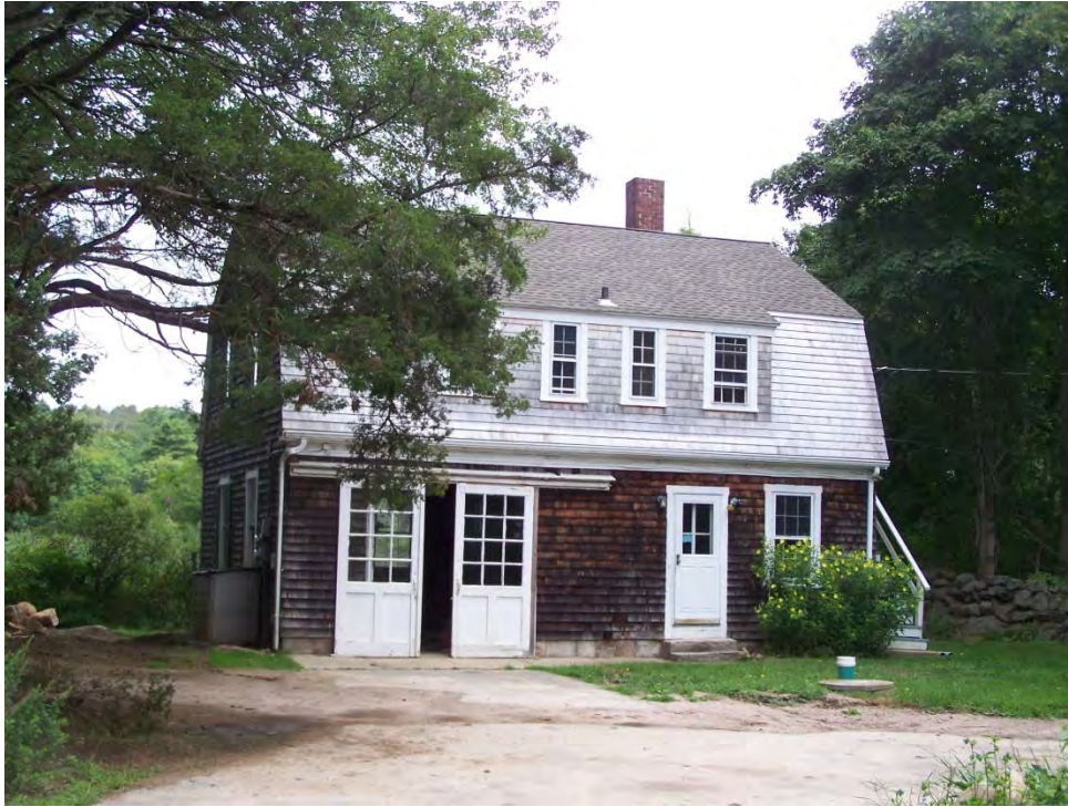
Ram Point Carriage House, before renovations, RCY 2013
