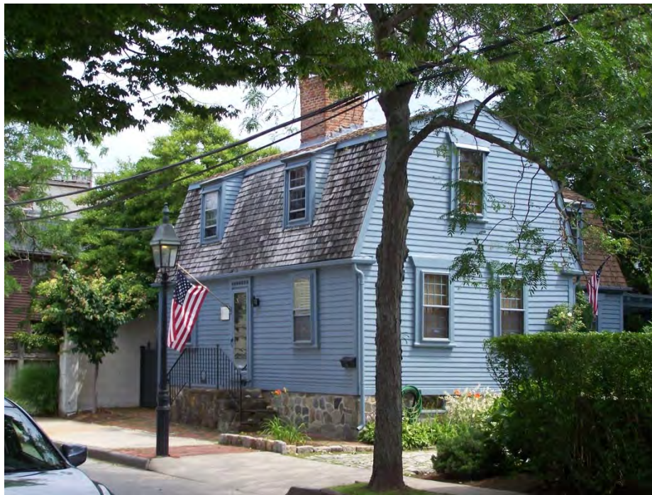
Bridge Street house, with existing raised foundation, looking west, RCY 2015
