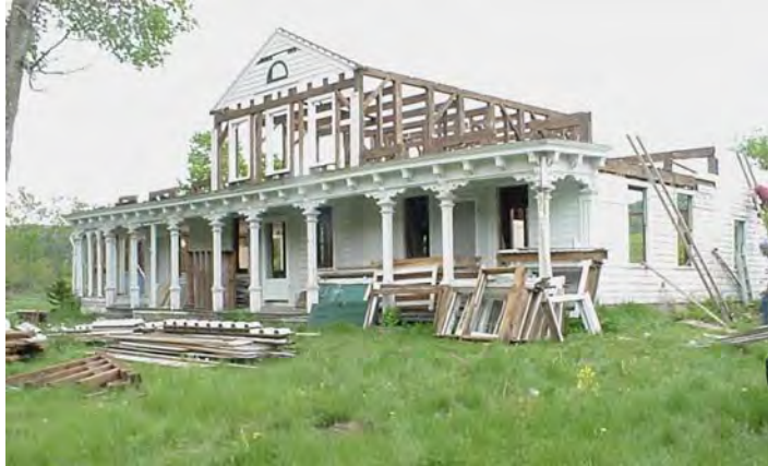
Dismantling of Bruchmann residence, May 2000
