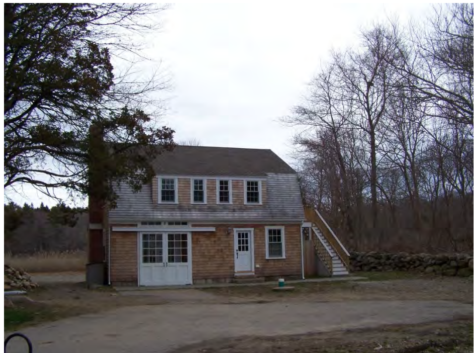
Ram Point Carriage House, after renovations, RCY 2015
