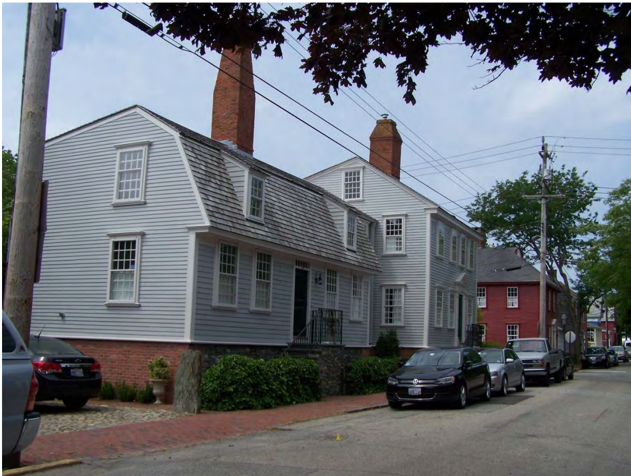
70 Bridge Street after rehabilitation with new raised foundation, looking west, RCY 2015
